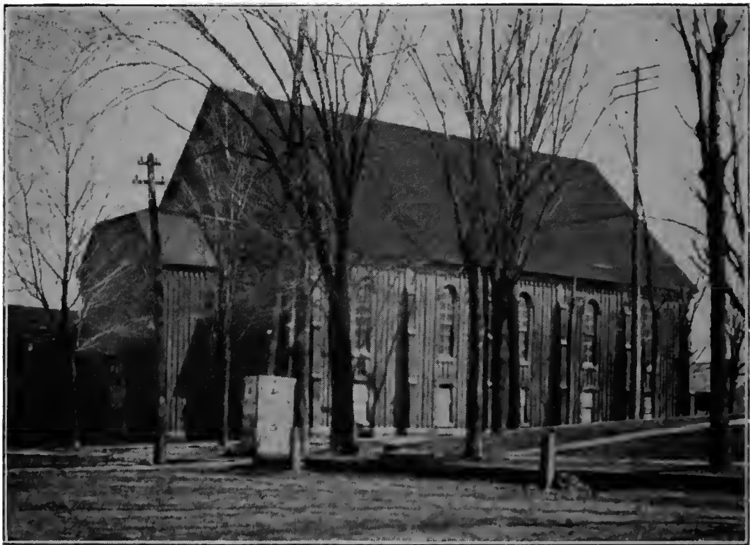
CONGREGATIONAL FREE METHODIST CHURCH Erected by L. Stiles, Jr., at Albion, N. Y., in 1858
